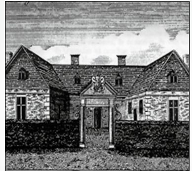
Old Men's Hospital
